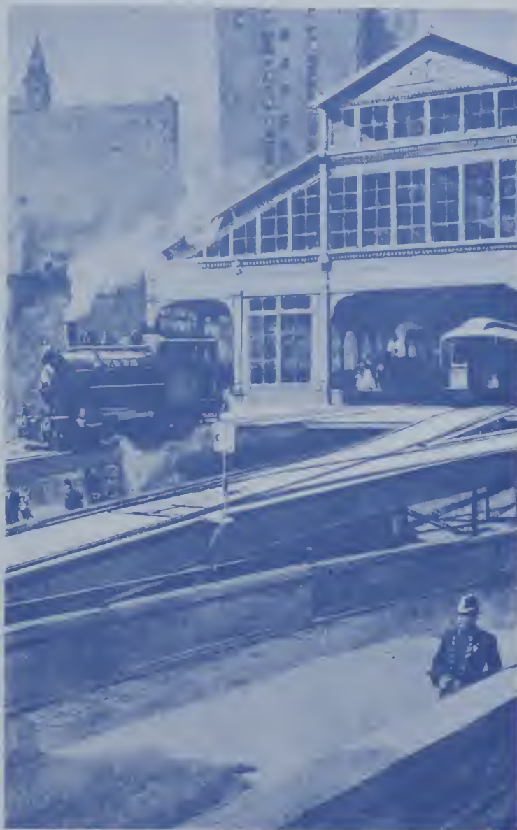
The Manhattan terminal of the bridge after reconstruction, which was started in 1893 and completed three years later. Trains were switched at the terminal by steam locomotives. After the cars were electrified, the locomotives were abandoned in 1897.
